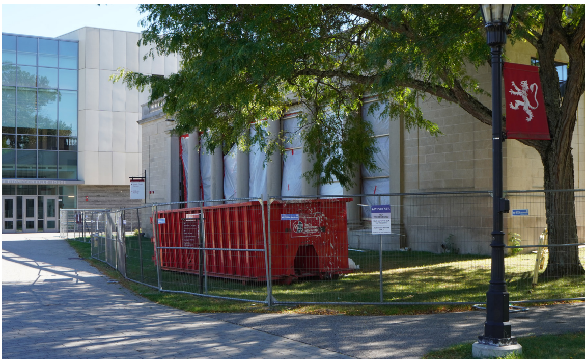
The Downer Fitness Center expansion is underway.
